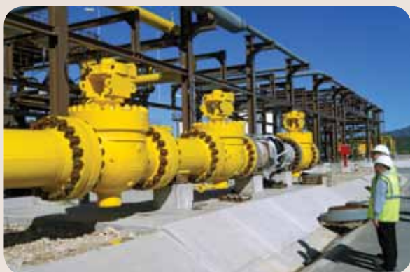
Onshore gas facilities
