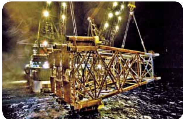
Installation of offshore platforms
