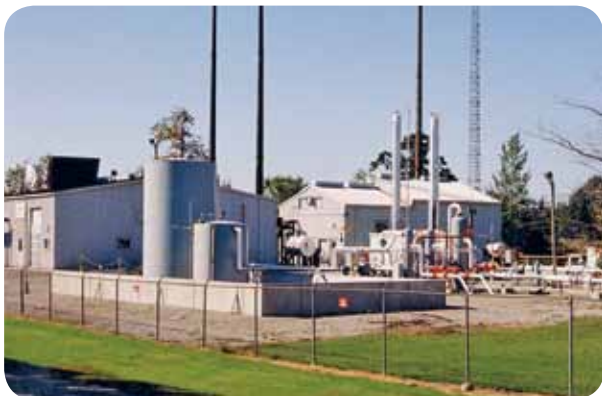
Port Maitland gas plant
