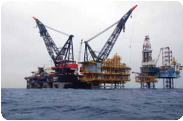
Installation of offshore platforms
