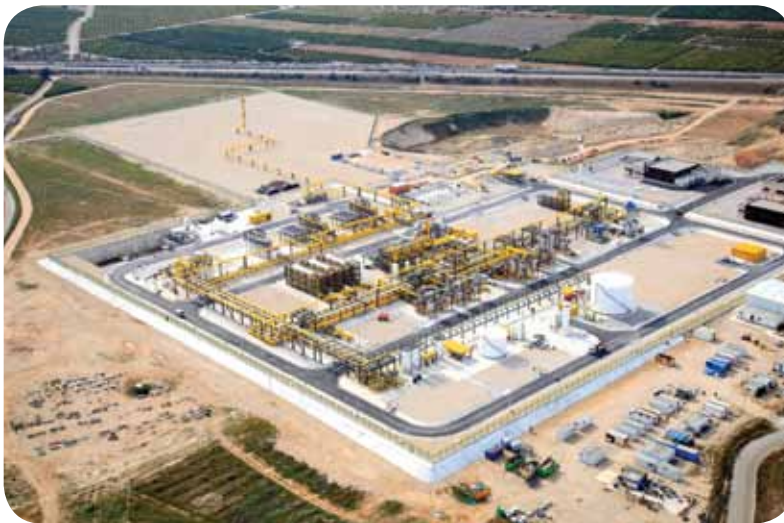
Onshore UGS facilities
